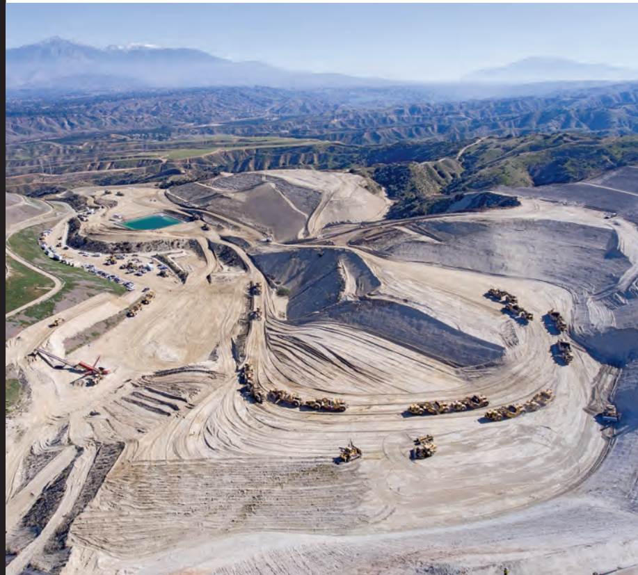
Sukut Construction ( No. 313 ) moves 2 million cu yd of material at a landfill excavation project in Redlands, Calif. Construction includes a desilting basin, two engineered stockpiles, 17 acres of composite geo-membrane liner, leachate collection and a stormwater system and paved haul road.
