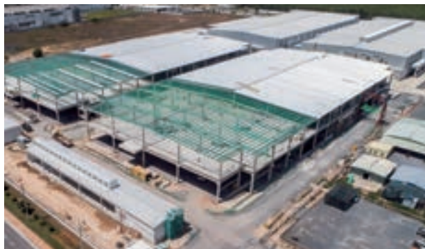
SMC Manufacturing (Vietnam) Factory No.2 (Second phase construction)
