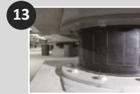
13 Seismic Isolation Bearings
