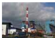
COAL FIRED STEAM POWER PLANT
