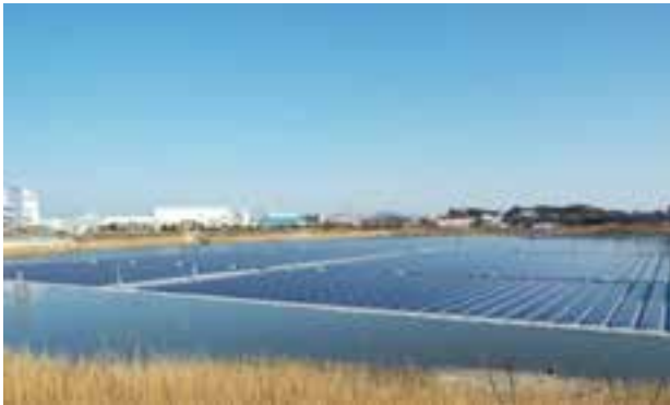
Water floating solar power generation plant (Certificated output:1.99 MW)
