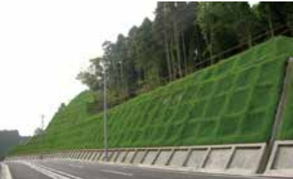
Slope constructed using the GT frame®
