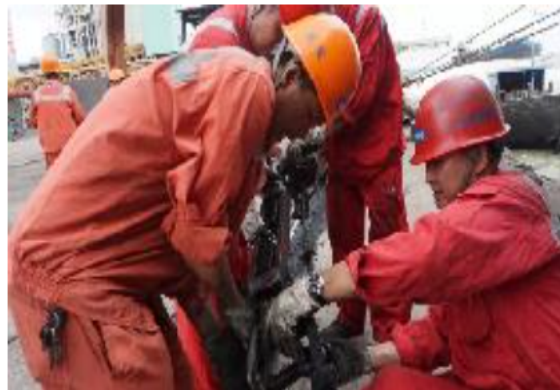
▲ Longwu Branch-reinforcing gantry crane
