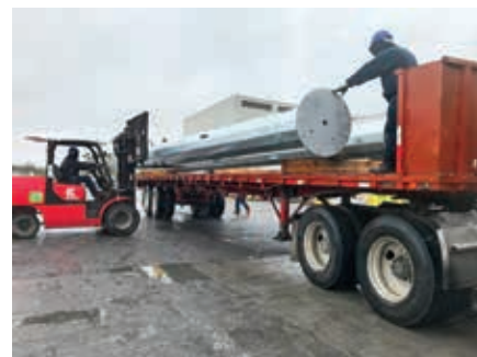
Dispatch of poles, SAE Towers
