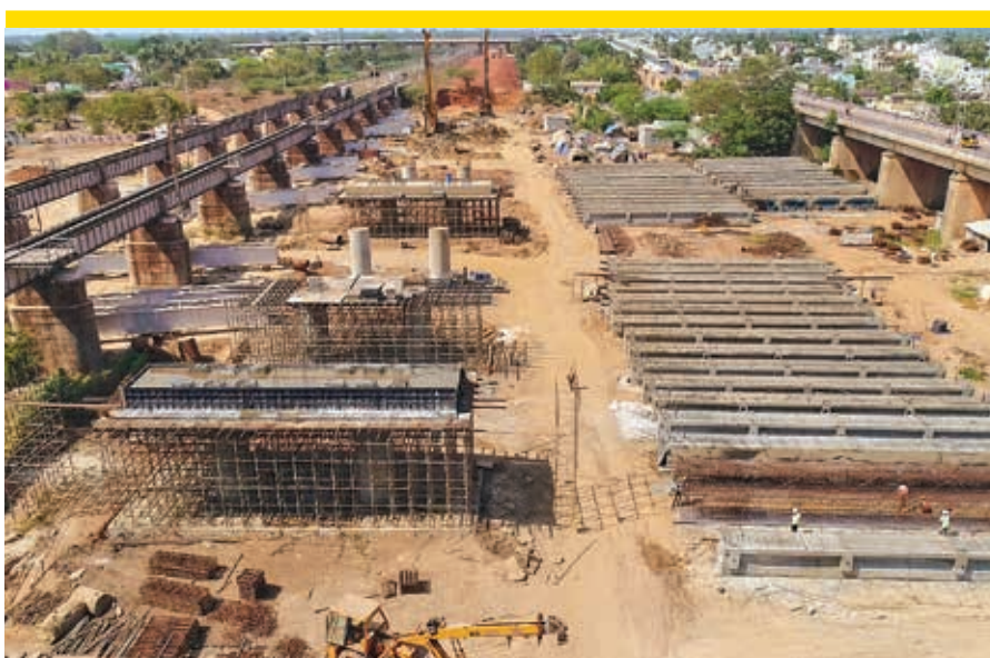
Work at major bridge across river Penna
