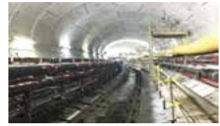
▲ Deep Tunnel Sewerage System Phase 2
