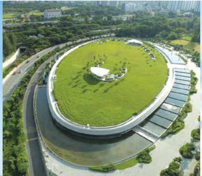
▲ Marina East Desalination Plant
