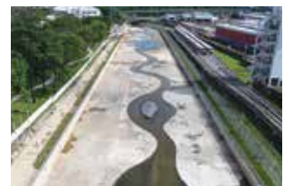
▲ Improvement to Kallang River
