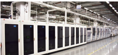
Power-on flow test
