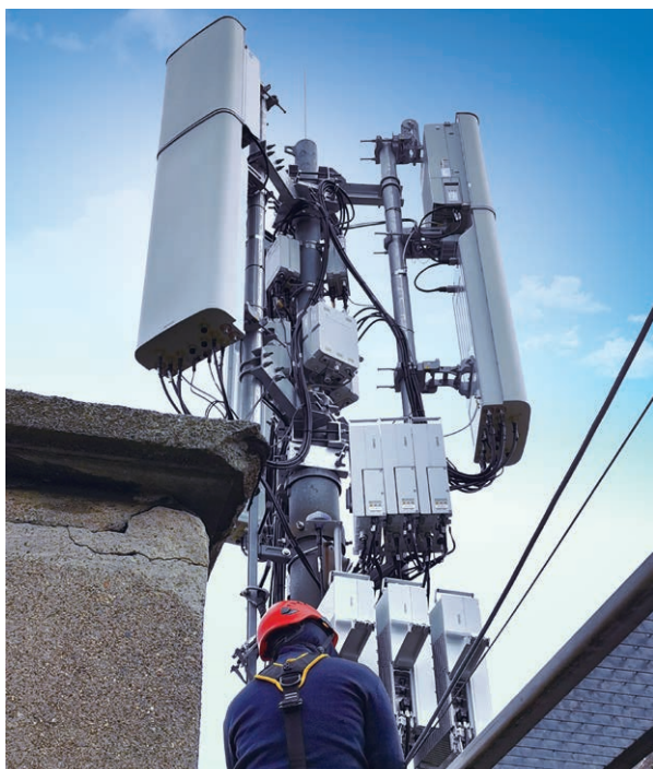
5G base station installation in Switzerland
