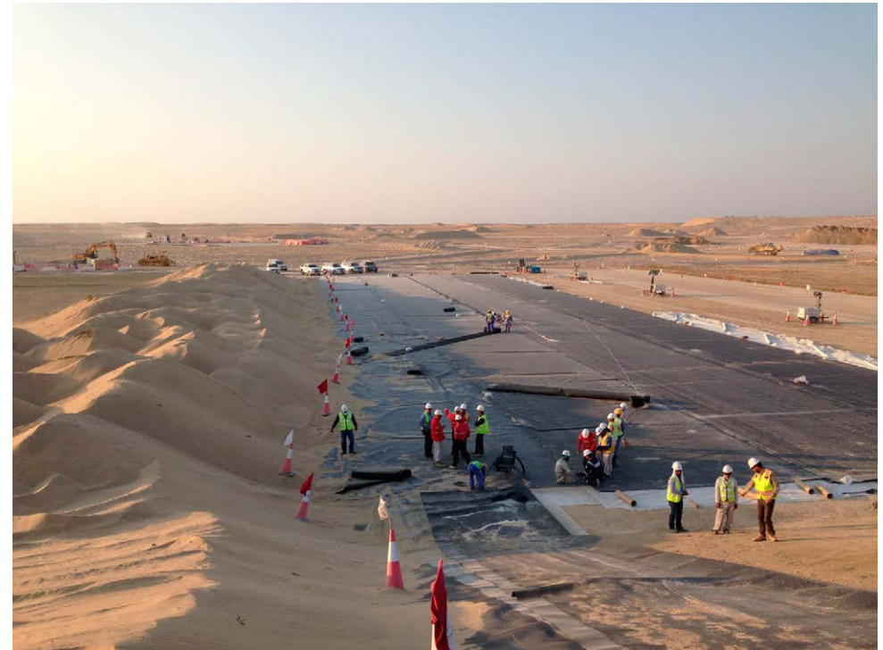
Initial stages of baseliner construction at Al Taweelah alumina refinery.
