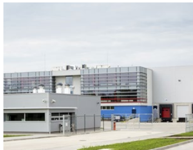
INDUSTRIAL AND MANUFACTURING
