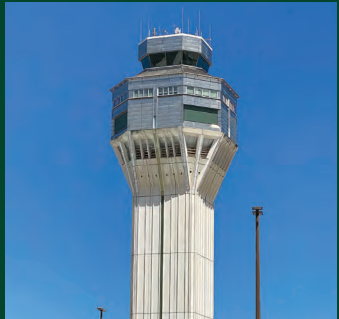
The San Juan Tower at Luis Muñoz Marín International Airport in San Juan, PR.
