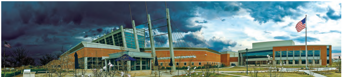
The David J. Hurley Air Traffic Control System Command Center in Warrenton, VA, which balances air traffic demand with system capacity. The Command Center is co-located with the Potomac Terminal Radar Approach Control, the facility in charge of the Washington, DC airspace.
