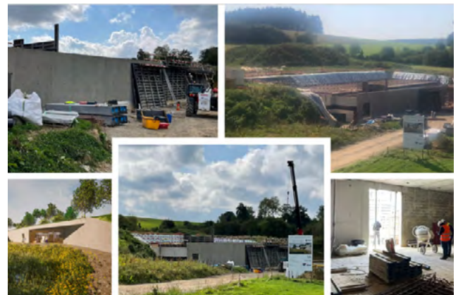
ECSC Construction site – November 2024
