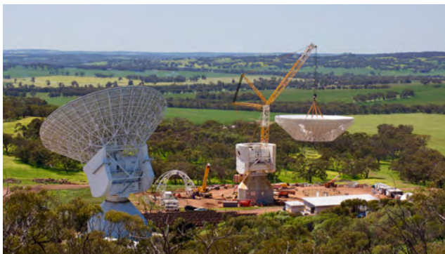
Lifting the dish at ESA's newest deep space antenna.
