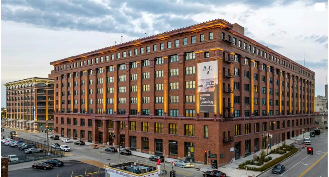
Guarantee Electrical played a key role in the renovation of the historic 735,000-square-foot Butler Brothers Building in St. Louis, now known as The Victor.
