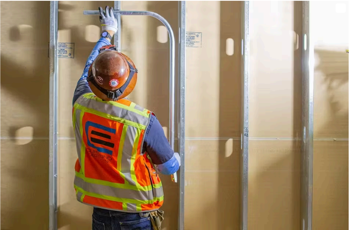
Cupertino Electric, Inc. (CEI) workers install electrical and low-voltage systems on this higher education upgrade project.
