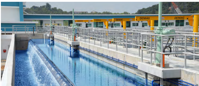
Langat 2 Water Treatment Plant constructed by MMC Engineering.
