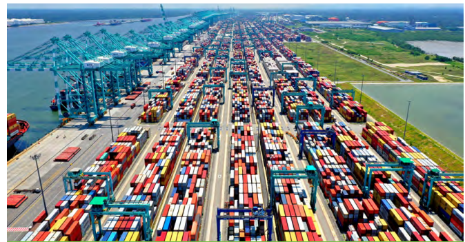
Aerial view of PTP's Container Terminal.
