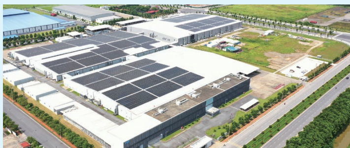
The YKK Vietnam Co., Ltd. Dong Van Factory (Phase 2, from the center-back section to the right-back section of the facility, has obtained LEED Silver certification)
