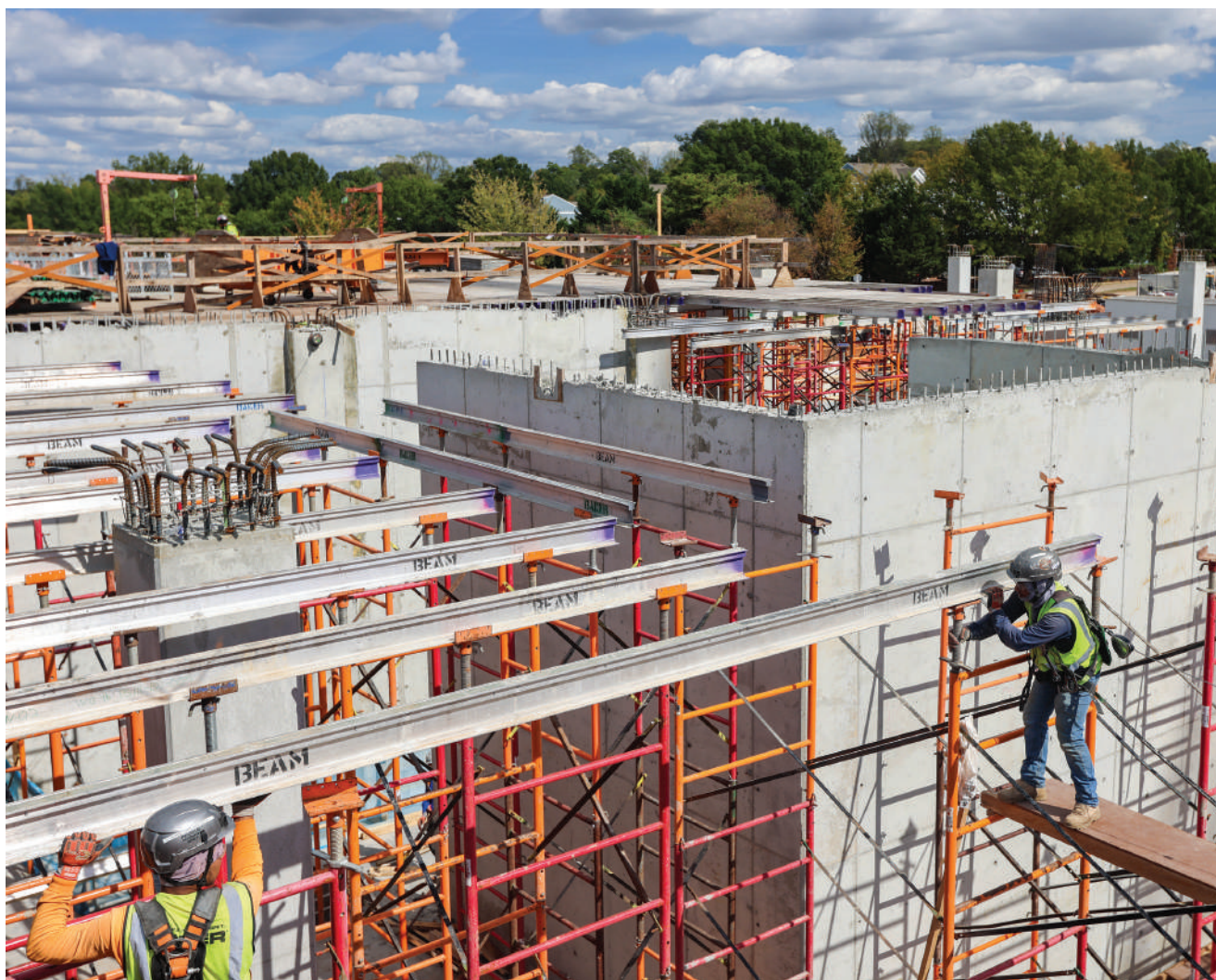
PHOTO COURTESY OF HITT CONTRACTING
